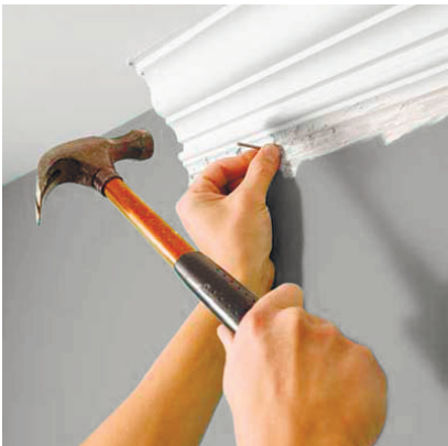
Ensure proper alignment on joints before nailing.
